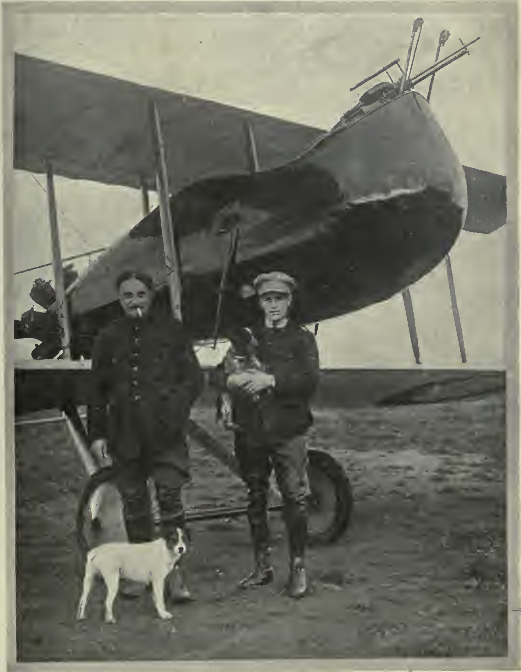
BELGIAN "PUSHER" MACHINE FITTED WITH LEWIS GUN.
