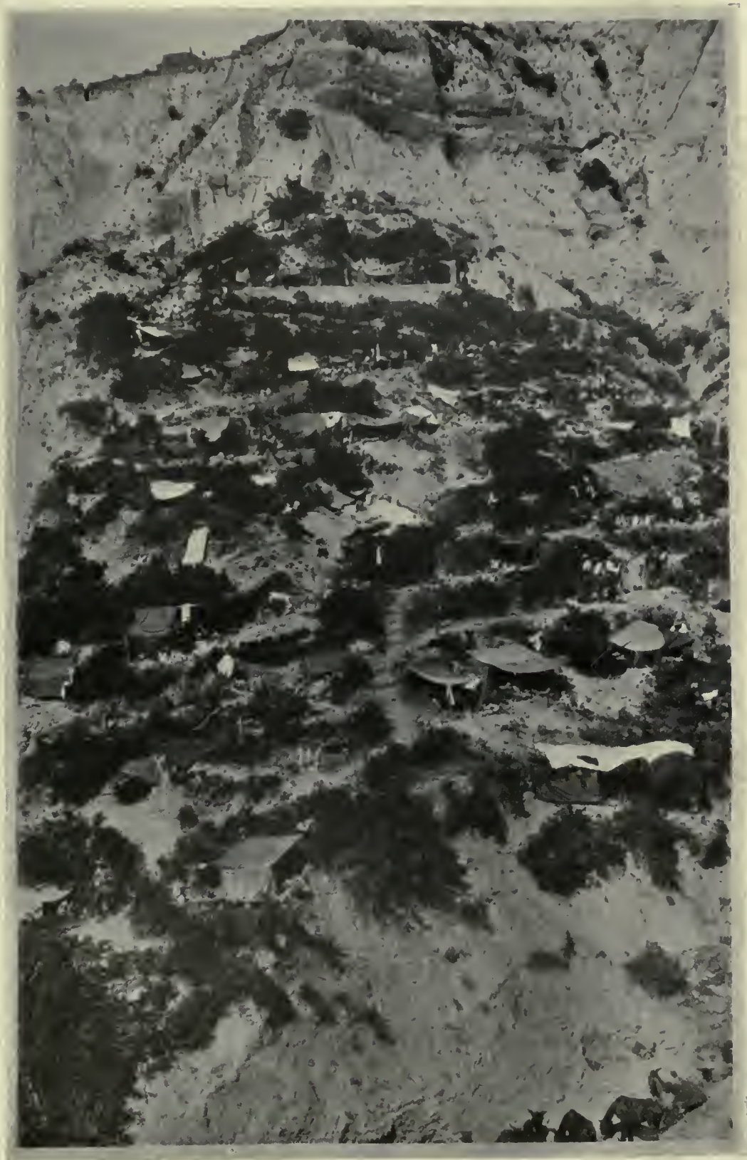
"DUGOUTS" CONSTRUCTED BY WELLINGTON MOUNTED RIFLES.
