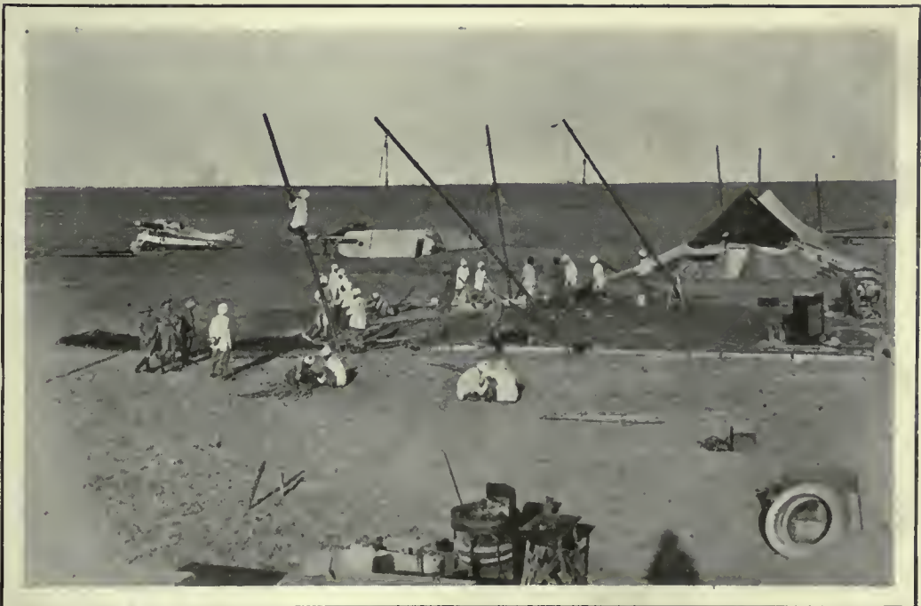
ERECTING PORTABLE CANVAS HANGARS IN THE DESERT.
