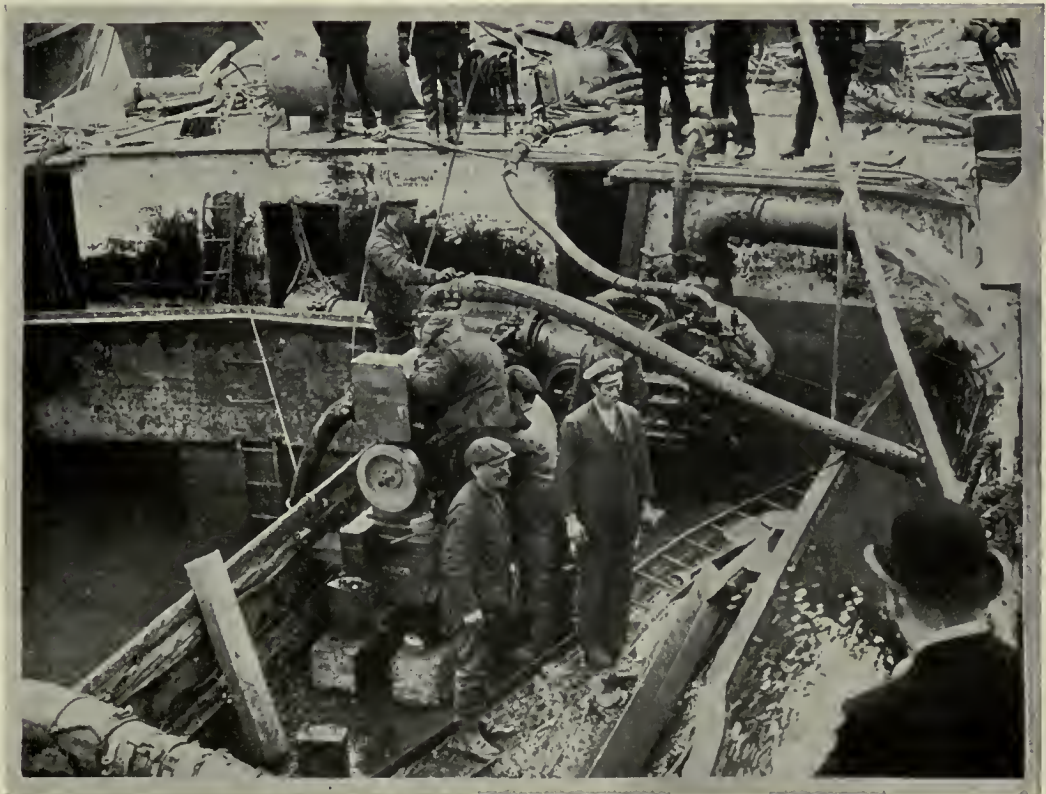
SALVAGE WORK IN THE NORTH SEA : THE PUMPING ENGINE.
