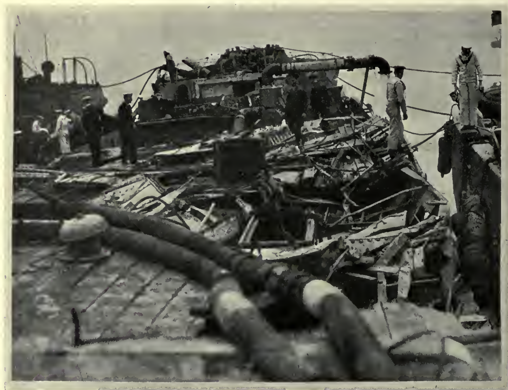
SALVAGE WORK IN THE NORTH SEA: PUMPING OUT A DERELICT.
