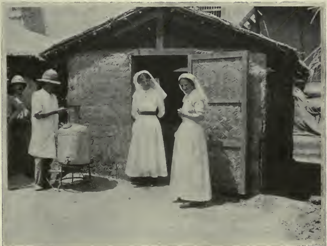
A HUT FOR DRESSING MINOR CASES AT AMARA.
