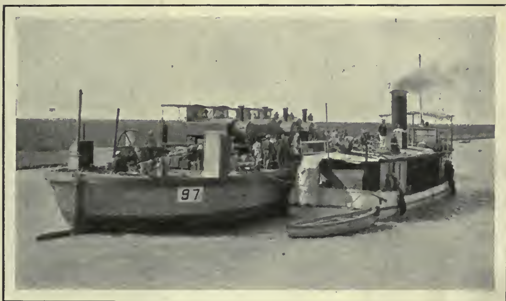
TRANSPORTING RAILWAY ENGINES UP THE TIGRIS.
